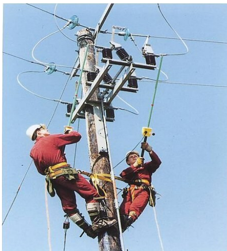
Overhead Line Testing
