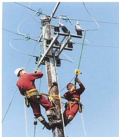
Overhead Line Testing
