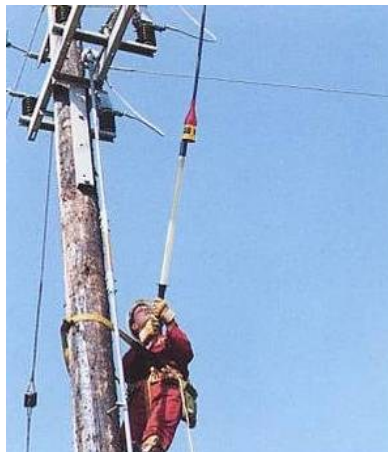
Overhead Line Testing
